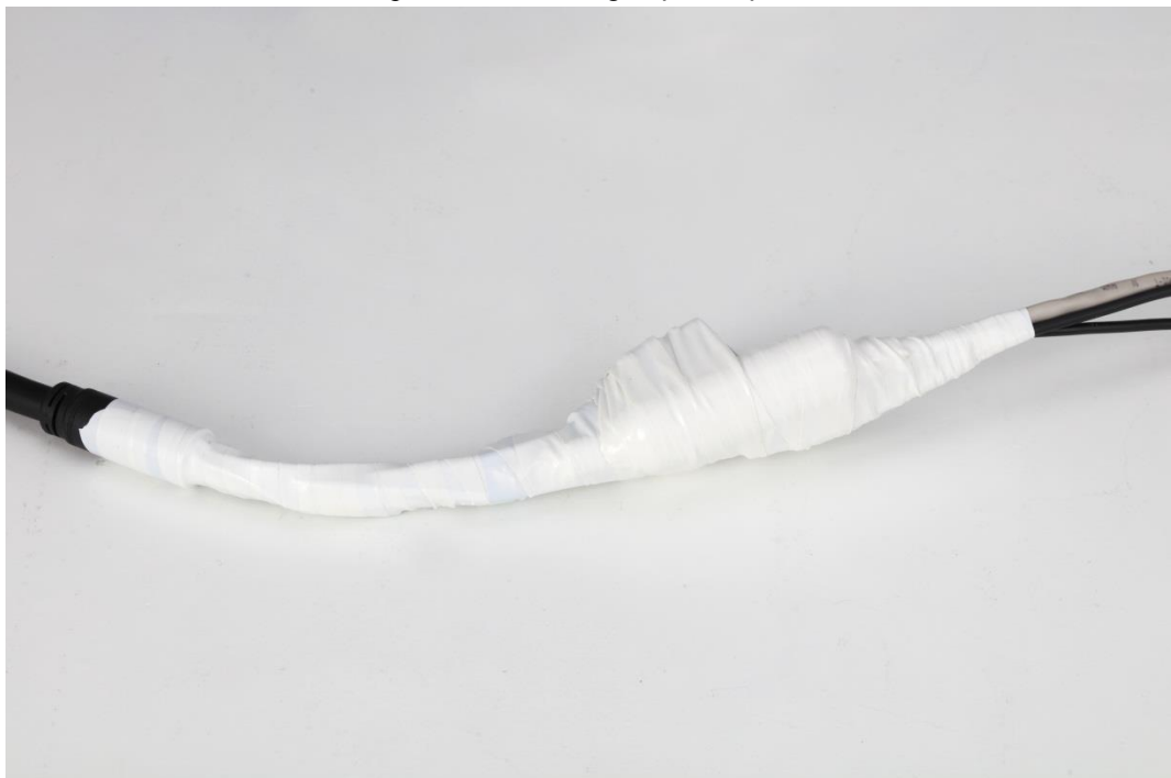
Figure 1-3 Covering exposed parts
